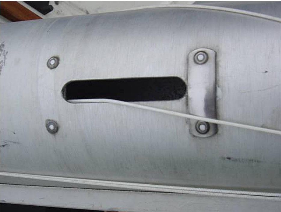
Slots for halyard exit from mast – S/S rounded bearing strips fitted internally & externally to prevent rope abrasion.
